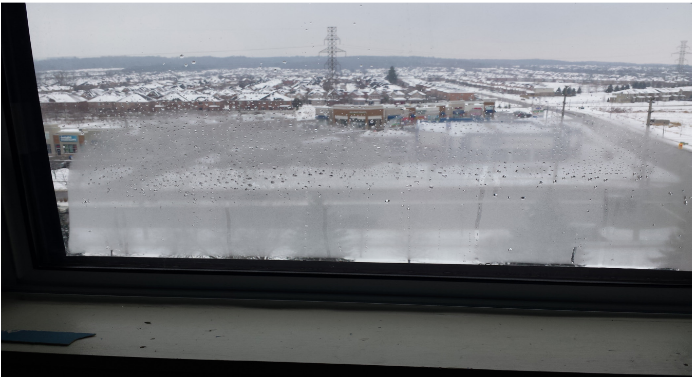
Condensation on an outer slider of a paired assembly, due to interior unit humidity.
