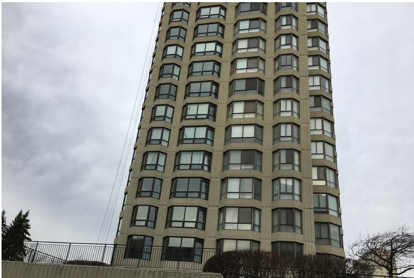
A window replacement project in progress. On the right are old windows, on the left are new ones. While they intentionally look architecturally similar, they are anything but, in terms of performance. Large, overhead paired, single-glazed sliders were replaced with fixed triple-glazed IGUs. Operable triple-glazed awnings were added in lower window areas. All IGUs were upgraded from double-glazed to triple-glazed, complete with argon gas fill and two low-emissivity coatings.
