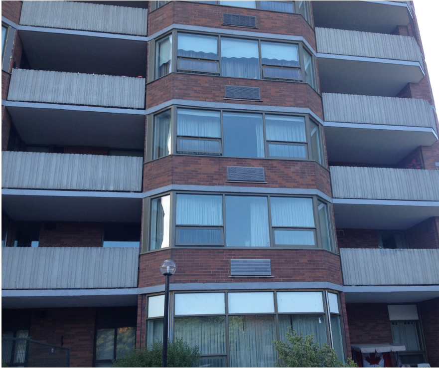
New, aluminum-framed windows with operable awnings for fresh air.
