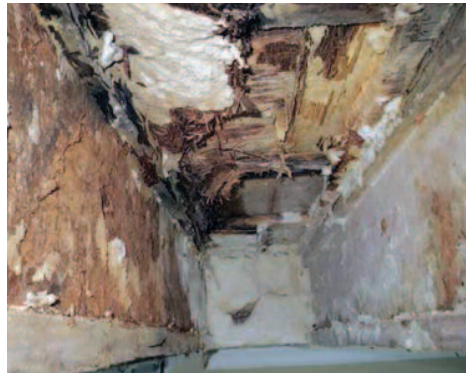
spray-foamed roof assembly may go unnoticed for years, allowing for significant deterioration of the structural framing.
