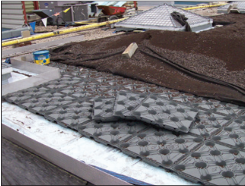
Laying the foundation for the green roof plants.
